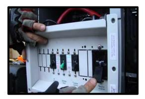
If your solar power inverter is more than 3 meters away from your switchboard, you must locate the switch marked, **solar AC isolator**. This will be located next to your inverter. If your inverter and switchboard are within 3 meters of each other, disregard this step.
