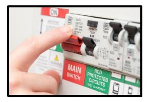
Go to your switchboard and open it. Locate the **solar supply main switch** and click the switch to the **off** position.
